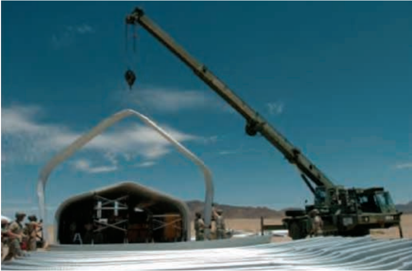
Combat Engineers from the 492nd Engineer Company from Mankato, Minnesota, use a crane to lift metal sheeting into place as they construct metal Quonset Huts at Forward Operating Base Miami on July 14th as part of Operation SAND CASTLE 2009. (Sergeant Brent Powell)
