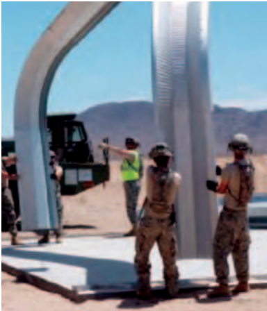
The 492nd Engineer Company constructs a Quonset hut on Forward Operation Base Miami for Operation SAND CASTLE 2009, at the National Training Center in Fort Irwin, California. The Soldiers are wearing the proper protective gear. (Staff Sergeant Raule Trado)
