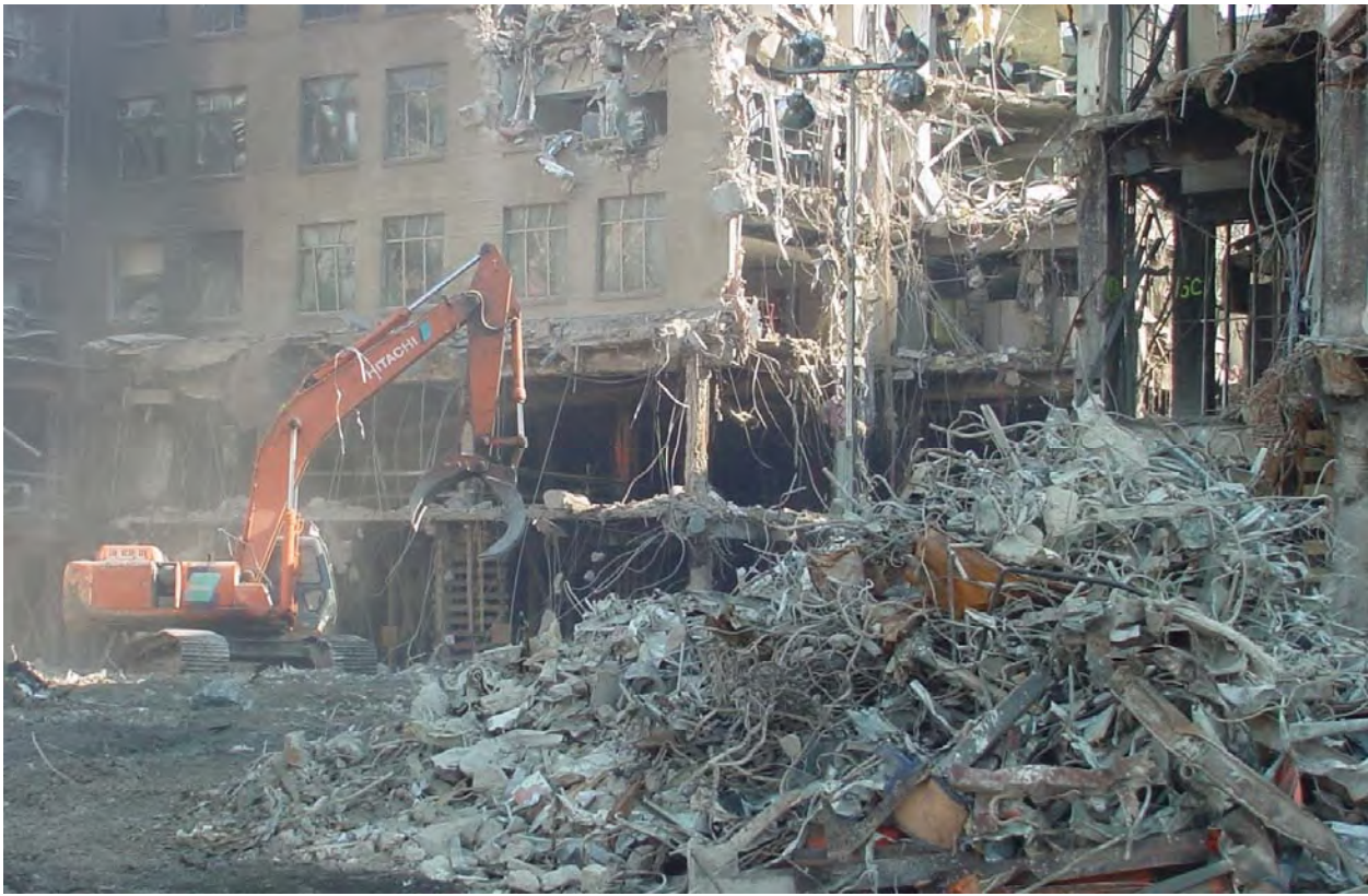
Arlington, VA, 22 October 2001 — An excavator uses a claw to tear down damaged sections and remove debris from the Pentagon. Rebuilding the Pentagon required that some damaged portions be torn down. (Photo by Specialist Kelly Strand, 46th MHD, Little Rock, AR).
