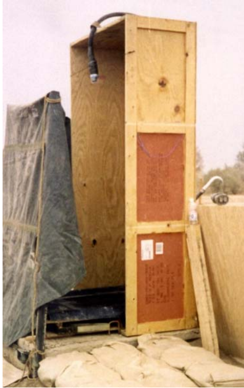
Showers were made possible through good old-GI-ingenuity: a barrel full of water, hand pumped through a hose to a makeshift shower head (a plastic Gatorade bottle punched with holes) draped over a makeshift plywood-and-canvas shower stall. Tallil, 2003.
