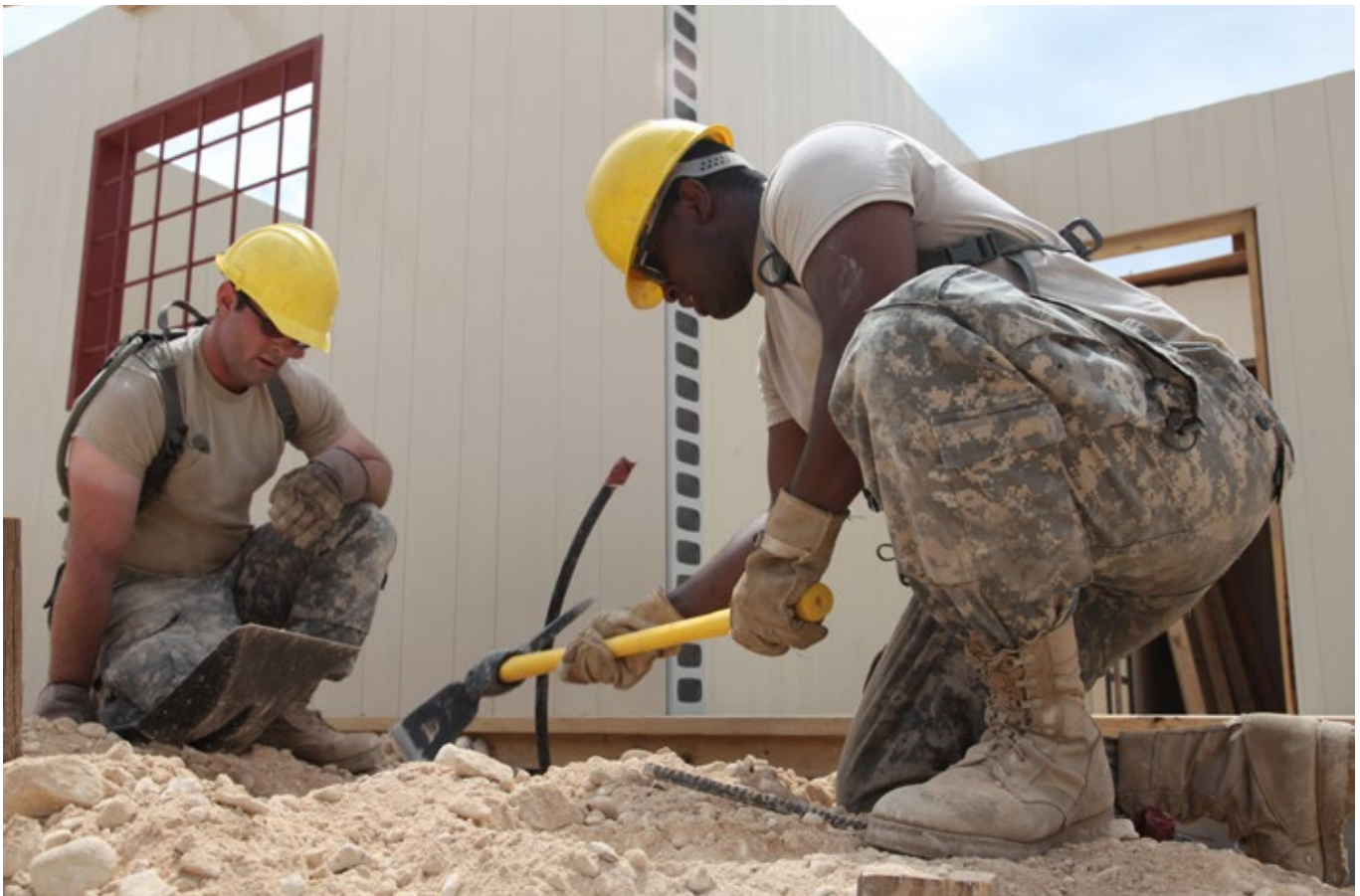
CONSTRUCTING HOPE. U.S. Army Reserve Soldiers with the 322nd Engineer Company from Decorah, Iowa, construct a medical clinic in Barahona, Dominican Republic during Humanitarian Civic Assistance Beyond the Horizon, May 2014. (U.S. Army photo by Sgt. 1st Class Bronco Suzuki/982nd COMCAM)
